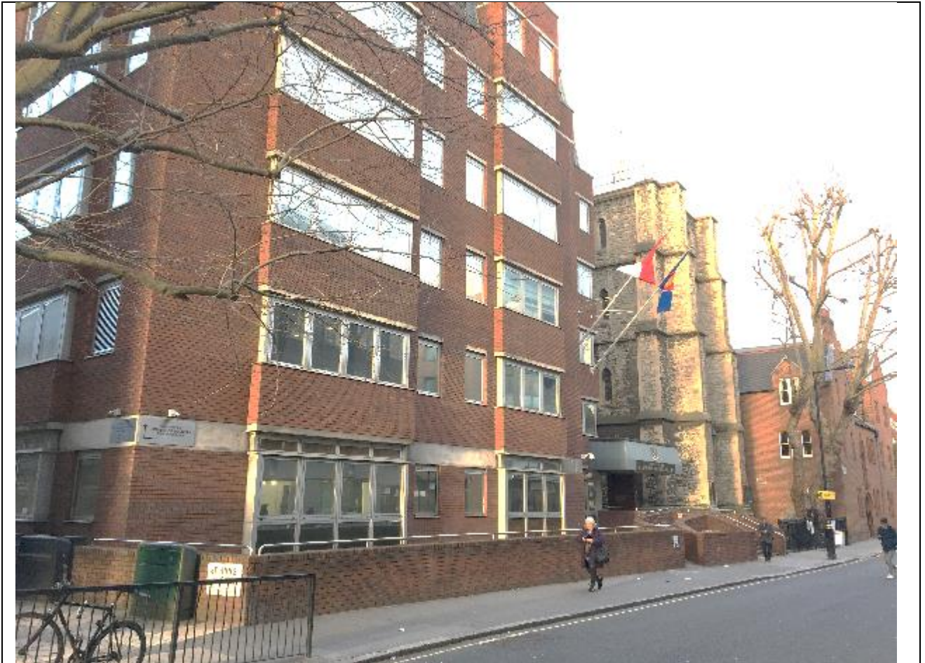
Photo 1: Front (south) elevation – site to left, St Matthew's Church to right.
